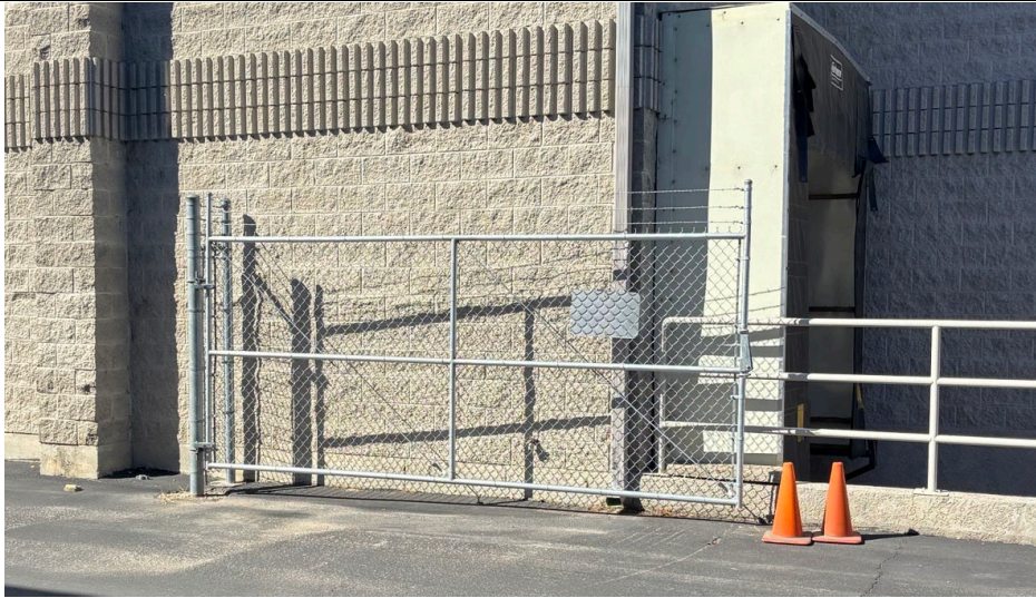
Figure 2. Shared Access Gate Constructed with Chain-Link Fencing and Barbed Wire
